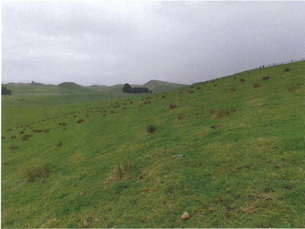
Figure A 4: Downstream face of the eastern embankment – looking south
