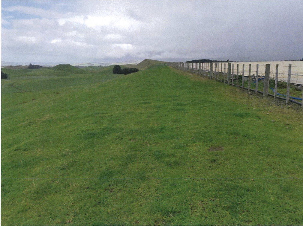
Figure A 5: Crest of the eastern embankment – looking south
