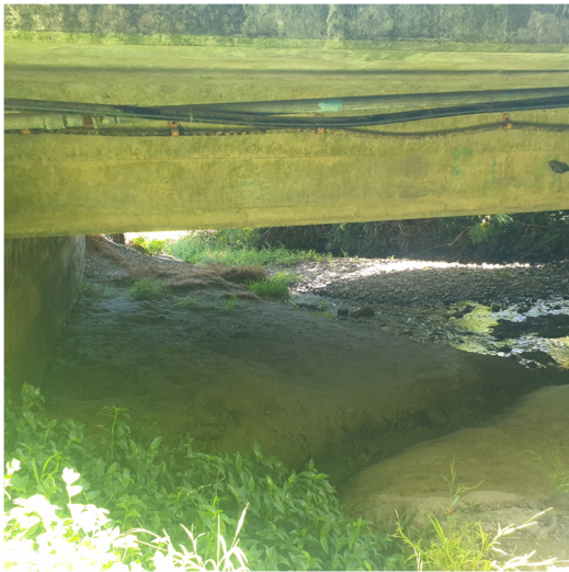
Looking downstream from under Victoria Avenue bridge
