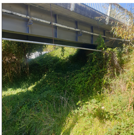
Under Cadman Road bridge, left bank
