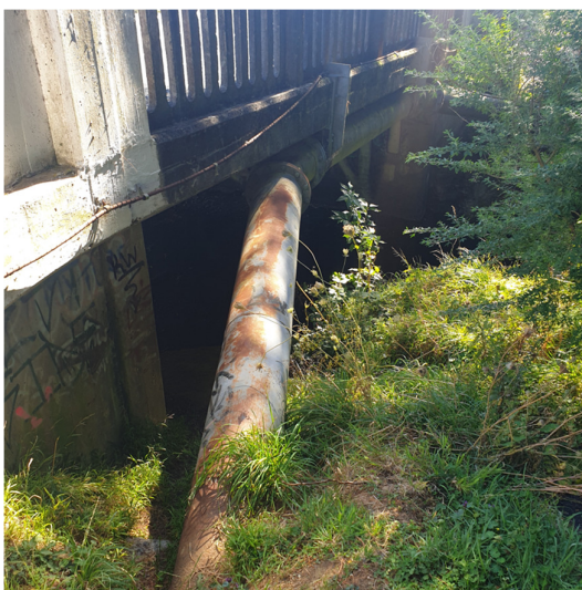
Cole Street bridge (upstream side)
