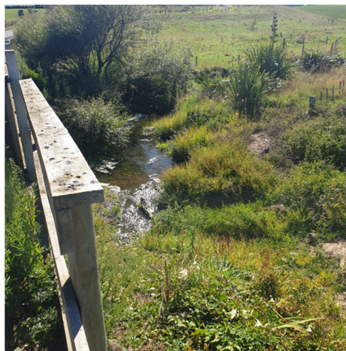
Smith Road bridge (upstream side)
