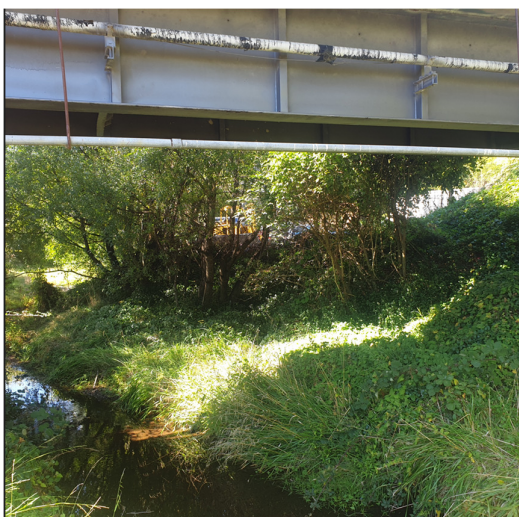
Looking upstream from under Cadman Road bridge
