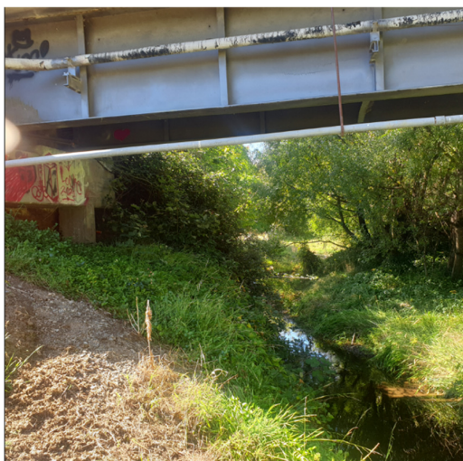
Looking upstream from under Cadman Road bridge
