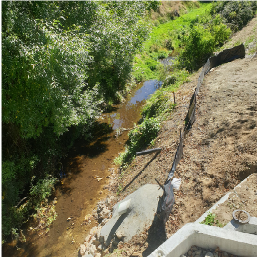
Looking upstream from Rawhiti Road bridge
