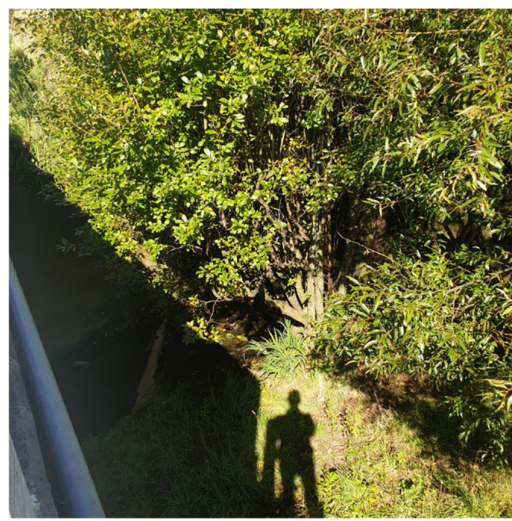
Smith Road bridge (downstream side)
