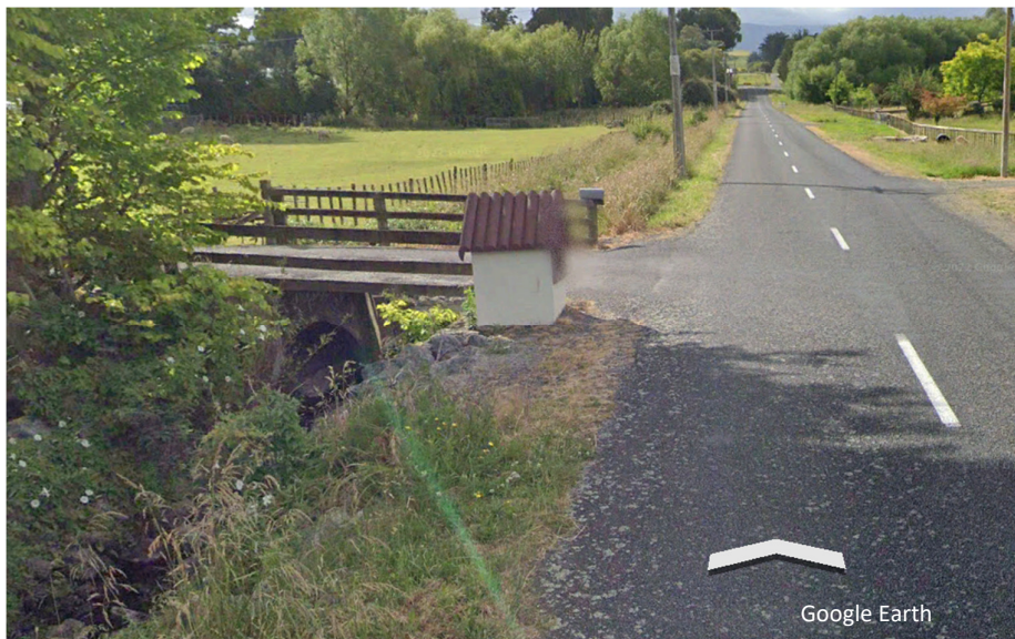
Figure 4-4 Culvert in drain, 109-111 Cole Street
