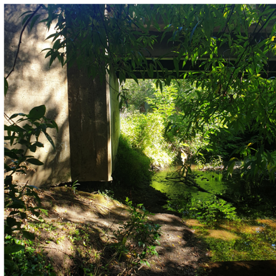
Looking downstream from under Princess Street bridge
