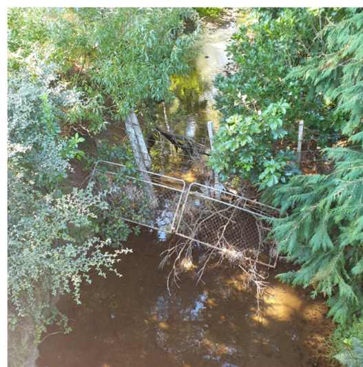
Looking upstream from Cole Street bridge
