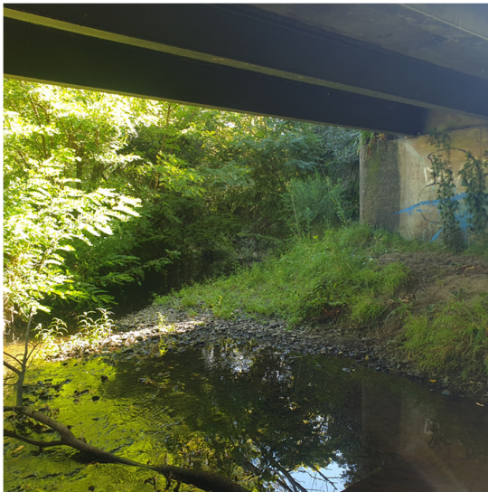
Looking downstream from under Princess Street bridge
