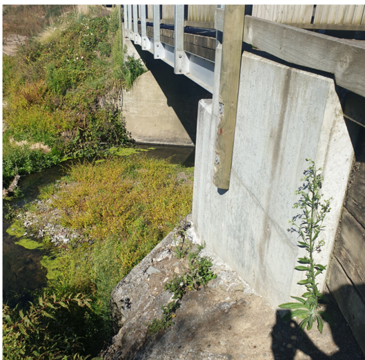
Smith Road bridge (upstream side)
