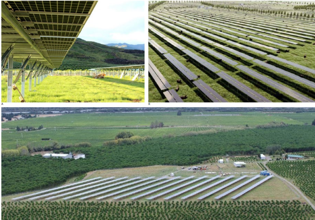
Figure 4: Example images of the proposed solar farm (taken from appendix 2 of the application).
