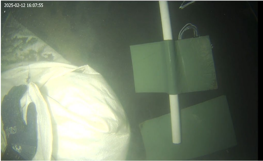
Depression 4 – Pinhole 2 repaired and marked.
